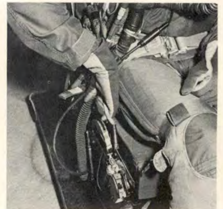
SURVIVAL KIT RELEASE HANDLE—ROTATE AFT.
